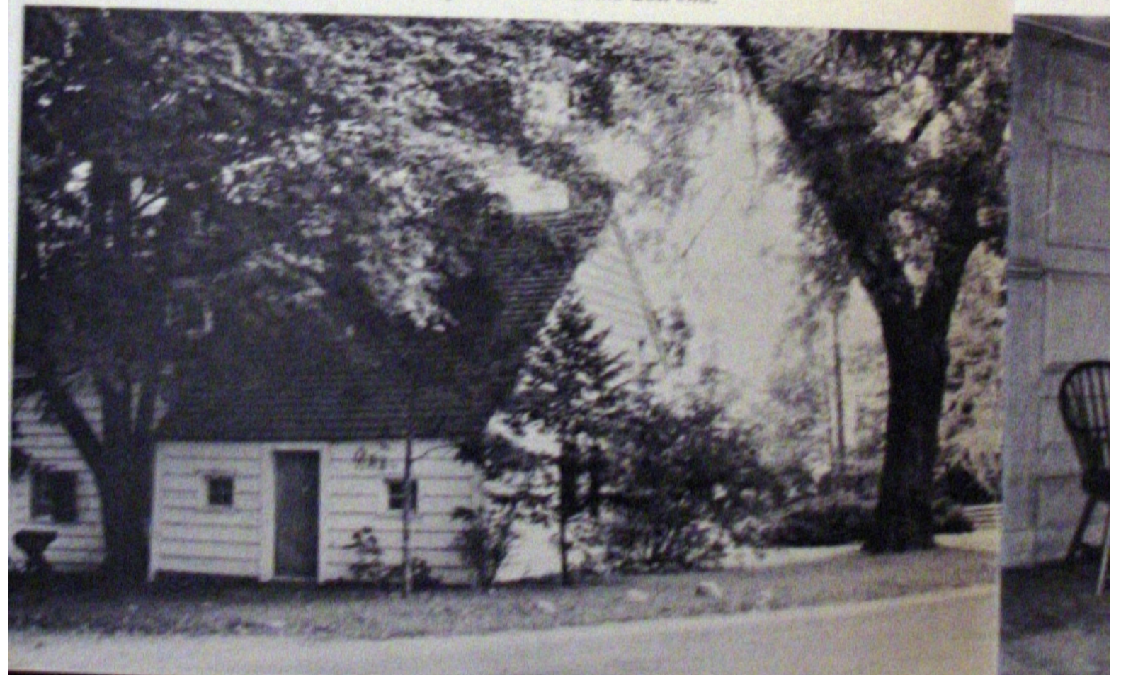
Rear of the little cottage which, almost as old as the Hammond home, was moved up and added at the west end.
